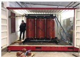
Manufacturer: Pauwels Type: Dry type 4500 kVA Rating: 20000 V Voltage prim.: Primary Tapping +/- 2x 2.5 % 400/231 V Voltage sec.: 50 Hz Frequency: Vector Group: Dyn 11
